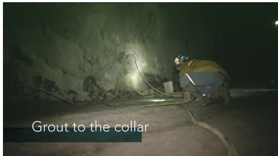
Figure 8 – Grouting MPBX
